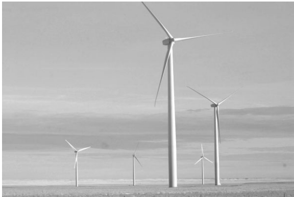
Figure 2 Wind energy turbines, like those pictured here in Judith Gap, Montana, can be 79.9 m tall with blades 38.4 m in length. At this size, the tips of blades can travel at up to 379.8 km h -1 . Often clustered to form 'wind farms,' these structures cause collision risk for a variety of avian species (Piorkowski et al. , 2012).
